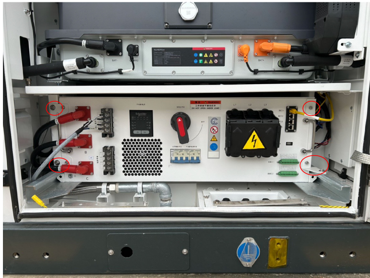
figure 5-20 Fixing screw schematic
