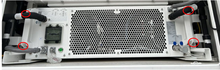
figure 5-29 Fixing screw schematic
