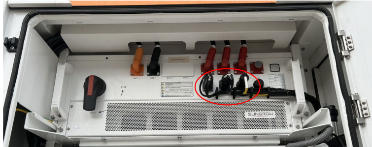
figure 5-23 Communication cable schematic
