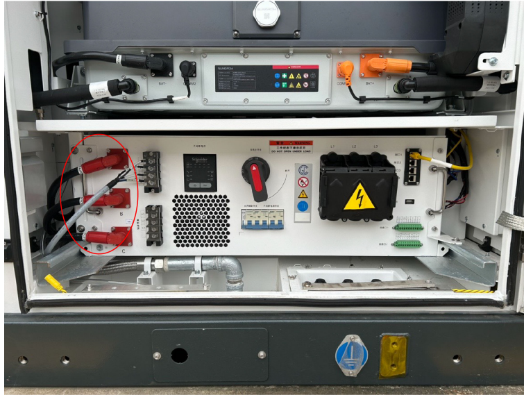
figure 5-15 Three-phase AC cable schematic
