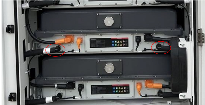
figure 5-14 Liquid Cooling Lines Schematic
