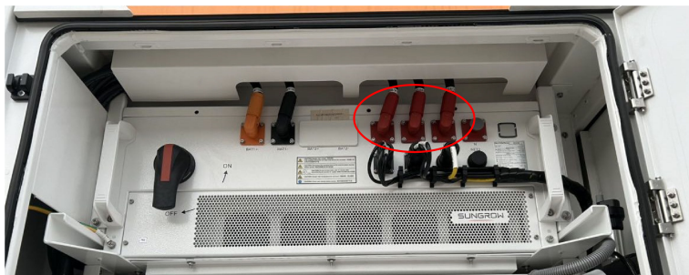
figure 5-22 AC side air plug schematic
