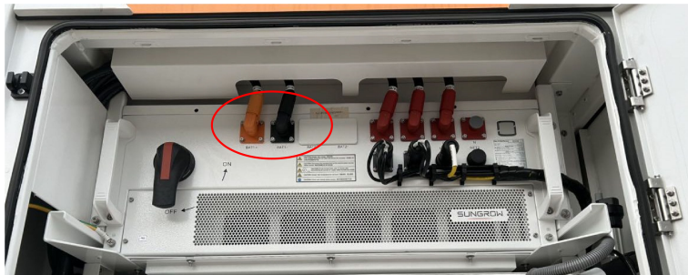
figure 5-21 DC side air plug schematic
