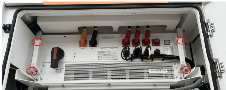
figure 5-24 Fixing screw schematic
