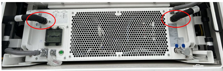
figure 5-28 Schematic diagram of inlet and outlet pipes
